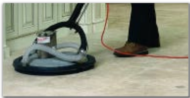
Tile and Grout
